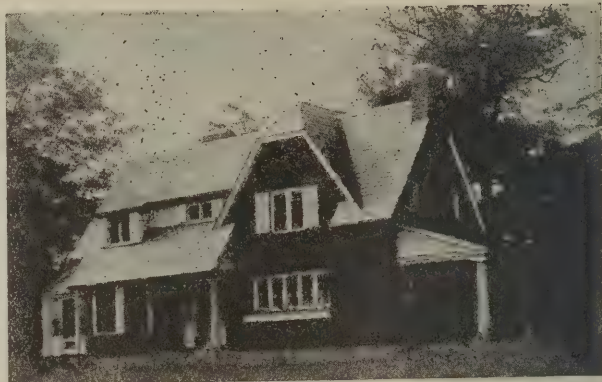
STRUCTURAL WINDOW BOX HARMONIZING WITH THE WOOD TRIM OF THE HOUSE. SHOULD BE SET LOWER, AS THE GROWING FLOWERS WILL LATER SHUT OUT AIR AND LIGHT FROM THE ROOM
